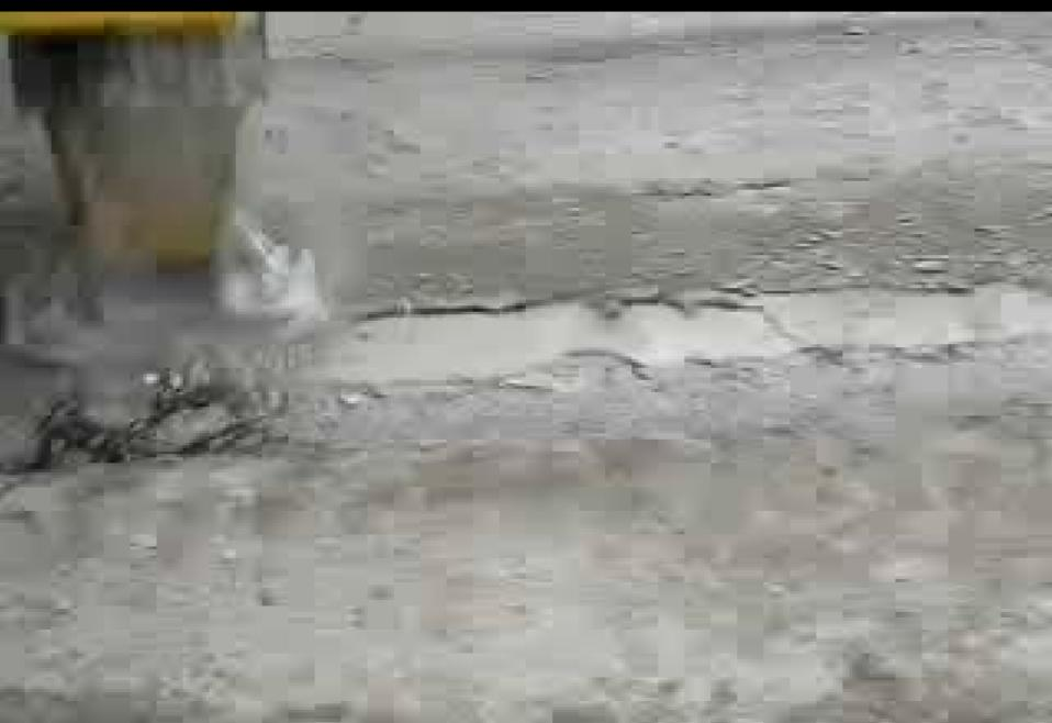
Test pits at WPAFB confirmed: - Complete slab destruction full depth (26 inches) - Nominal max particle size: 12 inches
